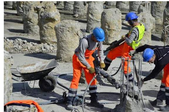
Breaking of Pile Head
