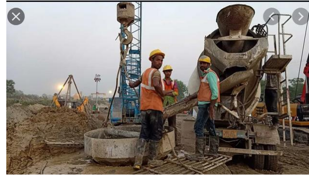
Pile Concreting
