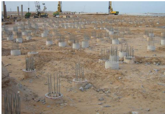
Piling work completed site
